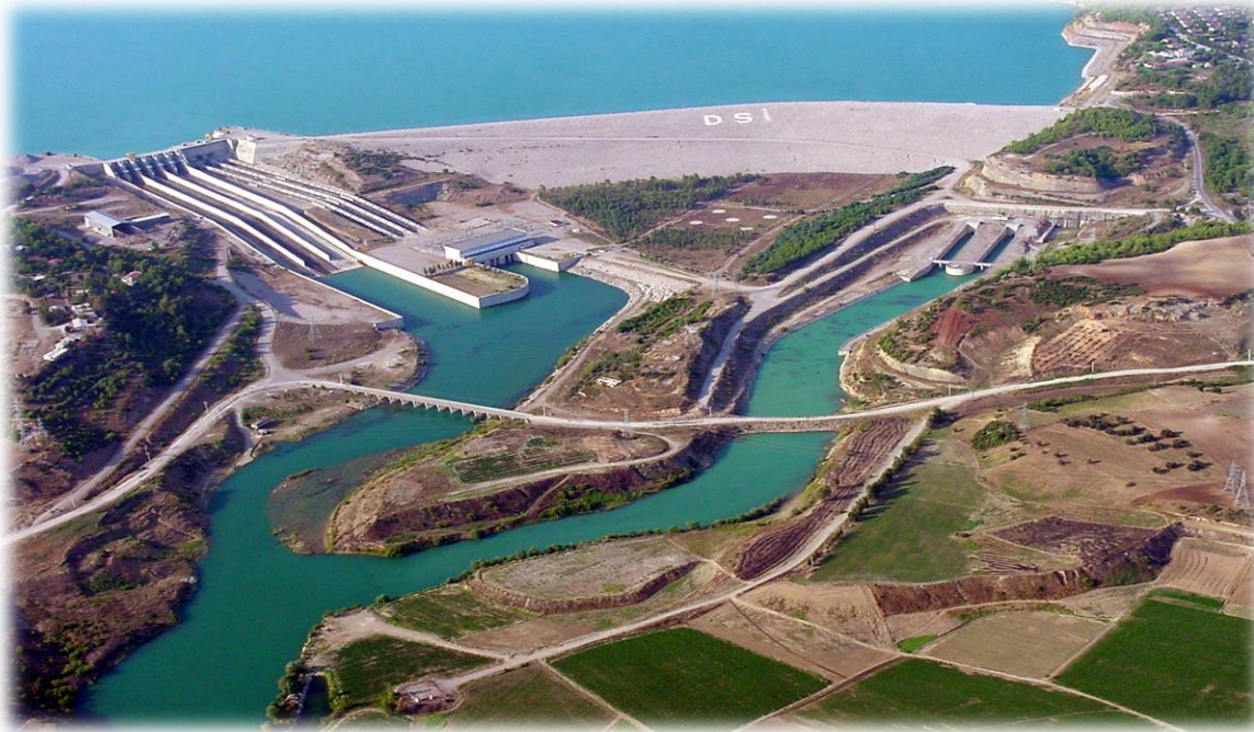
ÇATALAN HYDROELECTRIC POWER PLANT
