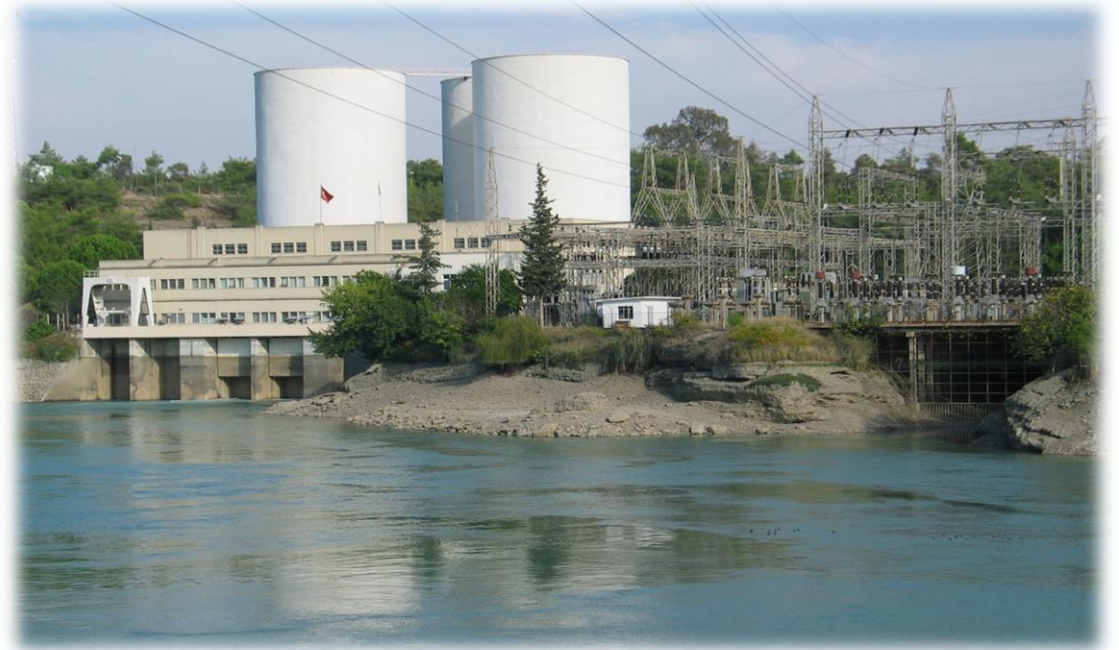
SEYHAN HYDROELECTRIC POWER PLANT
